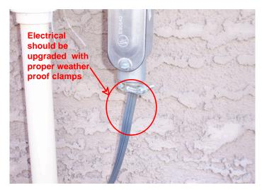
The outlet at the back patio extends away fromt the wall. Recommend repair by a licensed electrician
