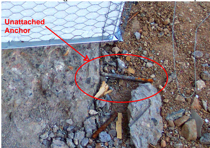
Figure Set - 8 The footers for the posts at the rear patio are in the process of being modified
