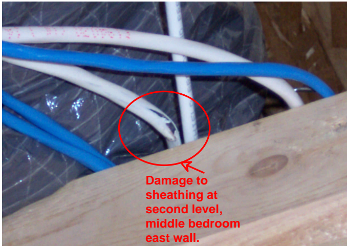
Figure Set - 16 The sheathing is torn on a section of the electrical cable
