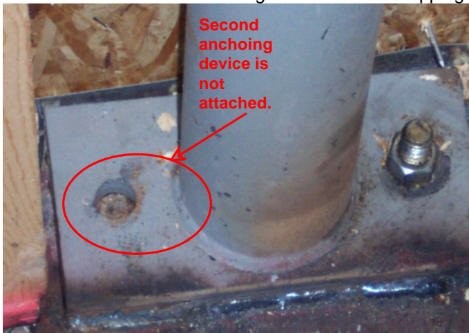
Figure Set - 6 The column supporting the bearing beam is not properly fastened to the foundation
