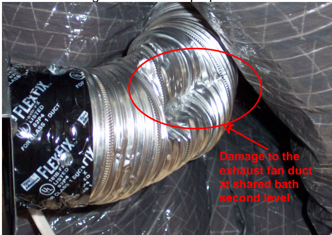
Figure Set - 14 The ductwork for the exhaust fan is constricted
