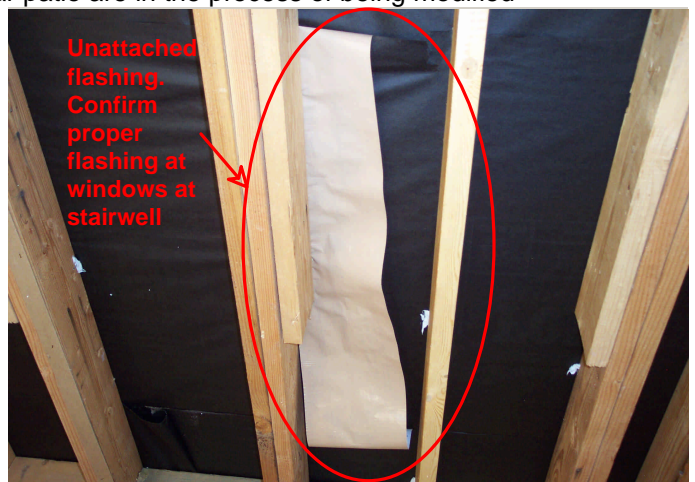
Figure Set - 9 The window flashing at various locations is not properly installed
