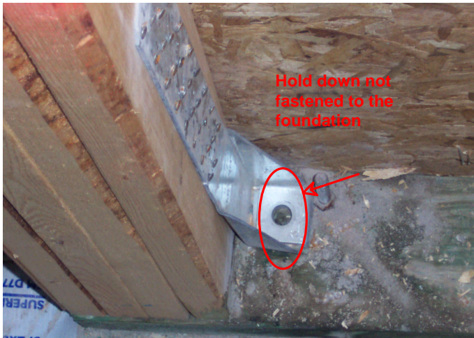
Figure Set - 1 There are numerous hold downs not fastened at the south wall
