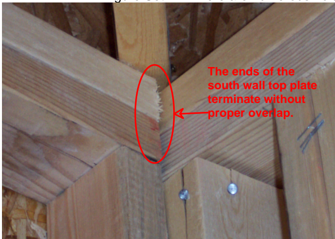
Figure Set - 2 The top plate must overlap at wall intersections and corners
