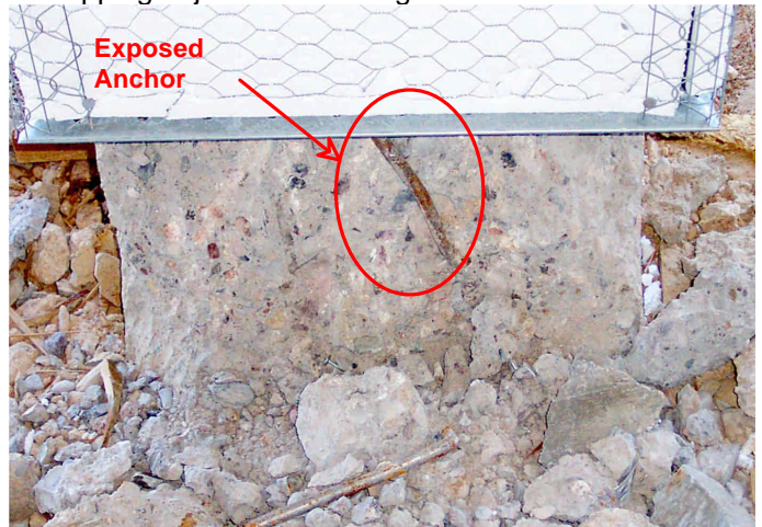
Figure Set - 8 The footers for the posts at the rear patio are in the process of being modified
