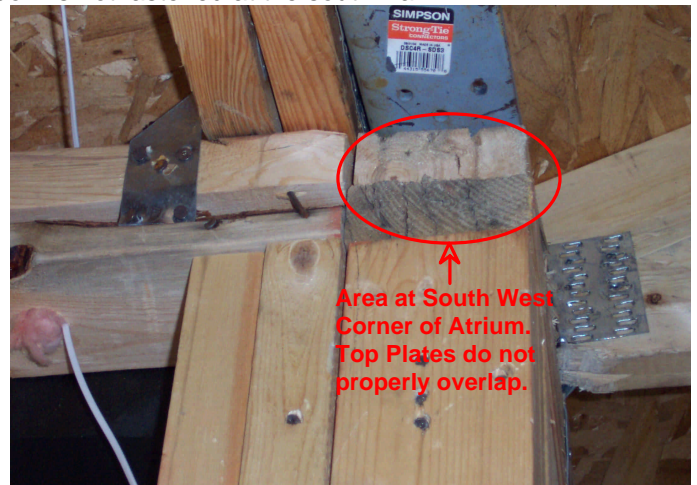
Figure Set - 2 The top plate must overlap at wall intersections and corners
